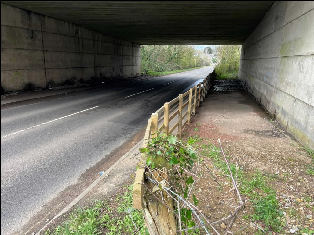
Photo 5-2: Existing Access Location (North) – Visibility (Looking Right)
