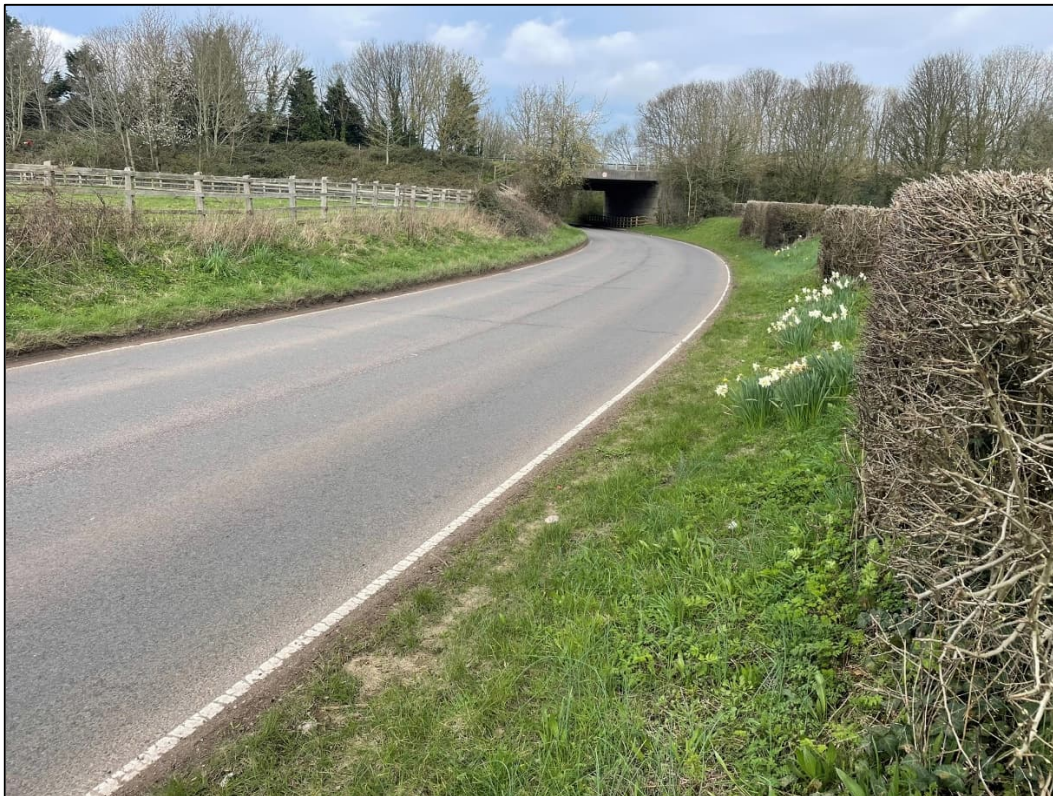
Photo 5-6: Alternative Access Location – Visibility (Looking Right)
